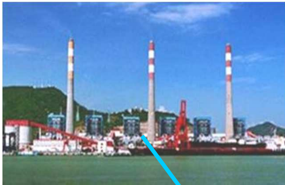
NSW FGD of Shenzhen power plant 6×300MW (1999 ~ 2004)
