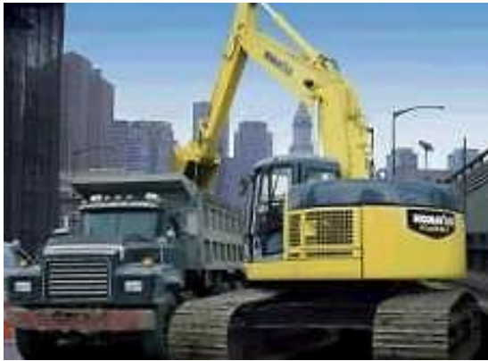
Road work in New York
