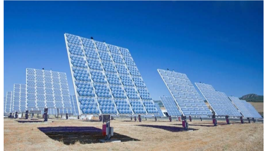
CPV: Lens array to focus sunlight on cells
