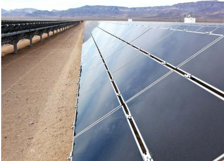
TF PV: Glass-on-glass laminates with Thin PV Coating
