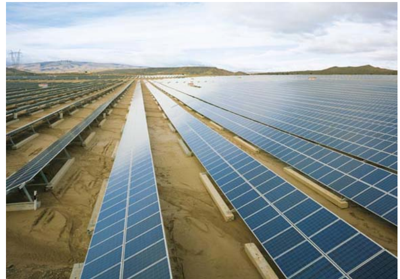
Crystalline PV: Si PV cells bonded on glass
