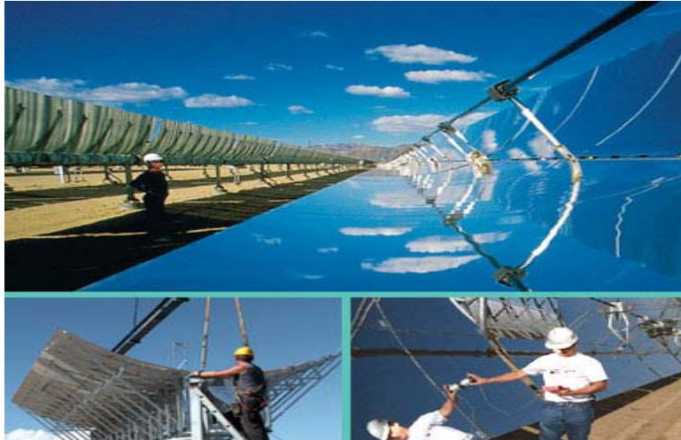
CSP: Tube of fluid heated by focused sunlight
